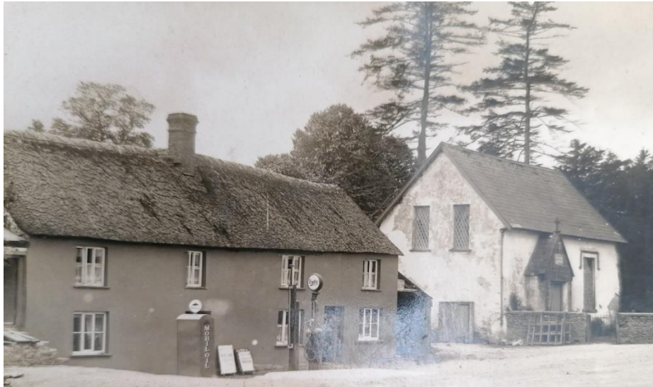
Hilary's family shop and the Church Room
