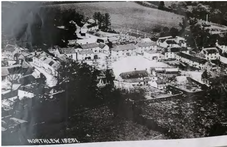
The Village - before all the parking.
